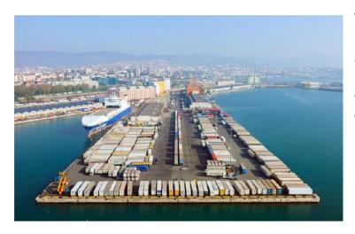
The Europa Multipurpose Terminal has an extension of **80.000 m2** and offers 1500 m of berths incl. landing place for Ro.Ro. ships. The terminal dispose on **4 rails** and **9000 m2 of warehouses**.
