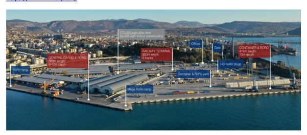
HHLA PLT Italy is a common user and multipurpose terminal located in the Customs Free Zone of Trieste's Ports and it has been operating Ro-Ro, Container, General Cargo, and Project Cargo since 2021. The terminal has two quays, for a total of 774m with a draft up to 13m, and the total area is 27 hectares with 65.000 sgm of covered warehouses and sheds.
