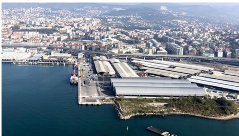
The General Cargo Terminal (148.000 m<sup>2</sup>) is focused on the traffic of wooden products and non-ferrous metals. The infrastructure disposes of one 350m long berth. The terminal has one rail track and is also provided with machinery for the **anti-stain treatment** of wooden products. At the terminal are at disposal ventilated warehouses as well as **30.000 m<sup>2</sup>** of covered surfaces.
