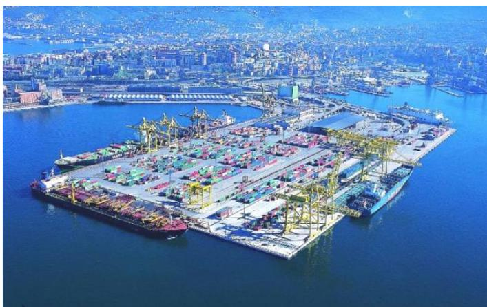
The TMT's container terminal has the **deepest natural draft of the whole Mediterranean Sea (18 meters)** at the berth), allowing all kinds of containerships to quickly and easily berth. The **5 rail tracks of 600 meters each** are served with 3 dedicated rail mounted stacking cranes. This modern infrastructure allows to manage **over 11.500 trains**
